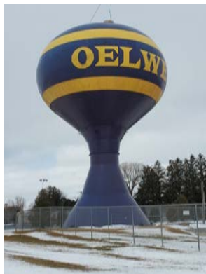
Oelwein Water Tower
