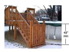
the gate must swing out and be self-closing and self-latching.
